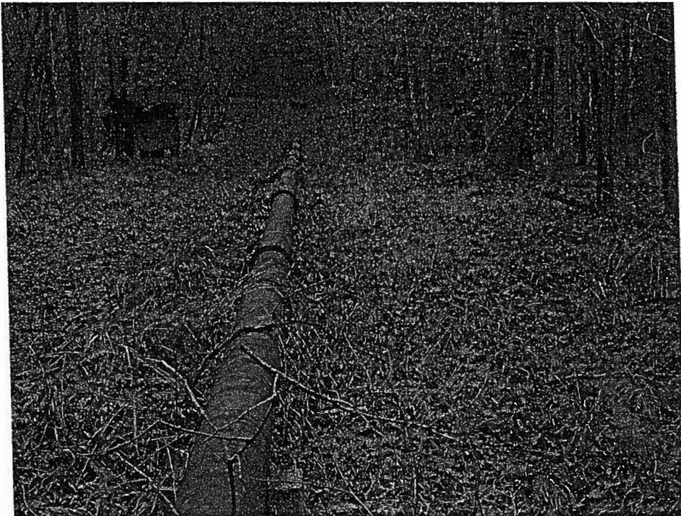
Exposed portion of sewer line ,
